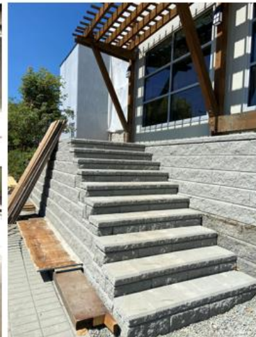
New emergency exit onto James Street
