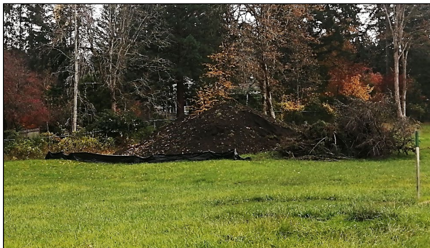
Photo 4: Soil pile has been seeded with grass seed to control surface erosion. Silt fence along toe of pile to prevent migration of fines towards the watercourse.
