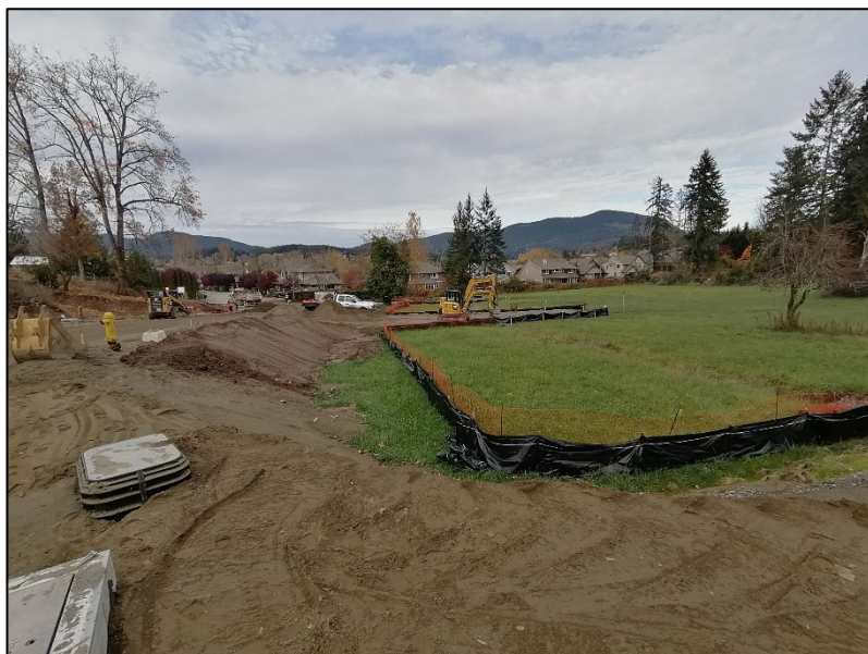
Photo 1: Looking north towards Trumpeter Close showing road construction underway and silt fence in place to protect the watercourse.
