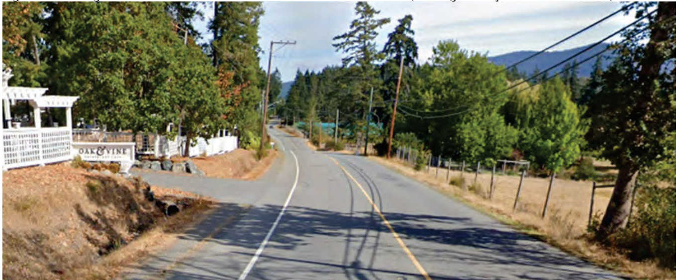
Figure 2: Existing Lakes Rd cross-section and access to 6380 Lakes Rd (looking north just south of access)
