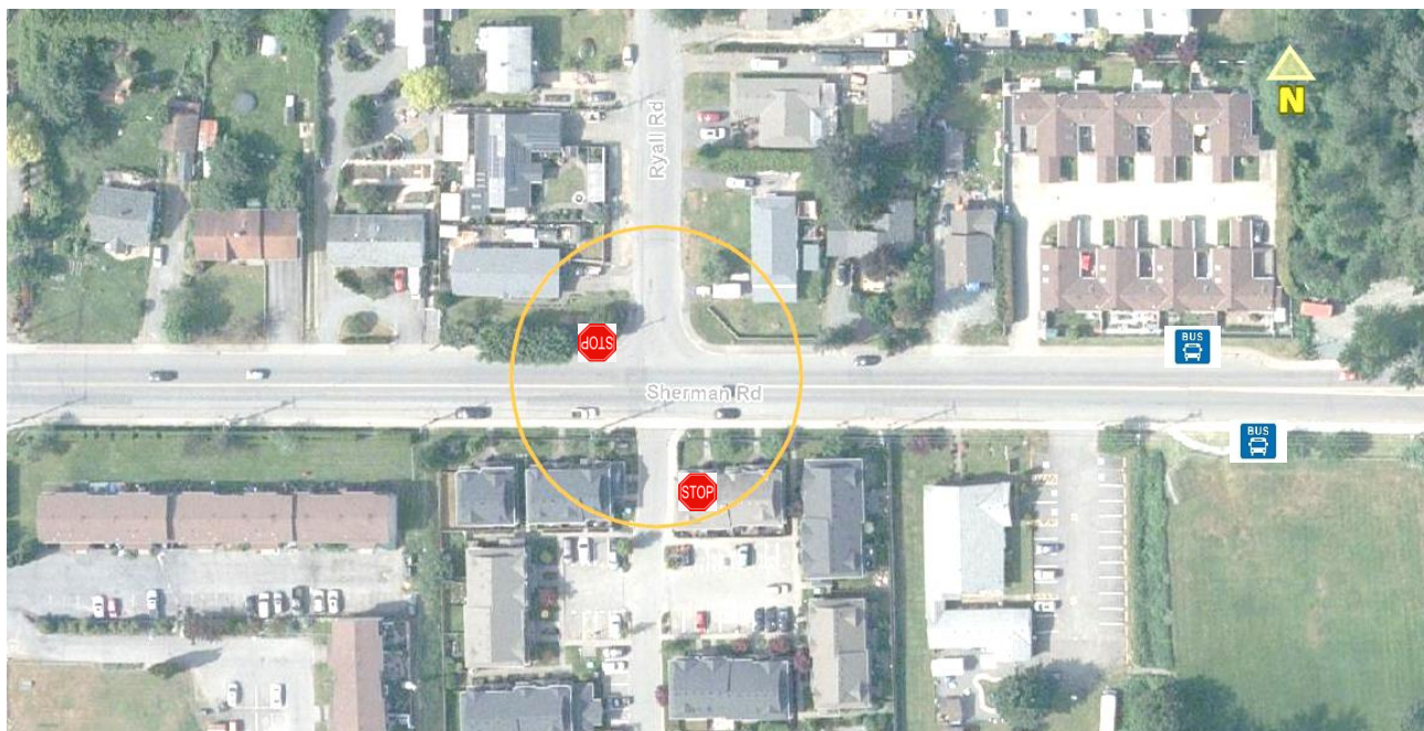
Figure 1: Site Location – Sherman Road/Ryall Road Intersection
