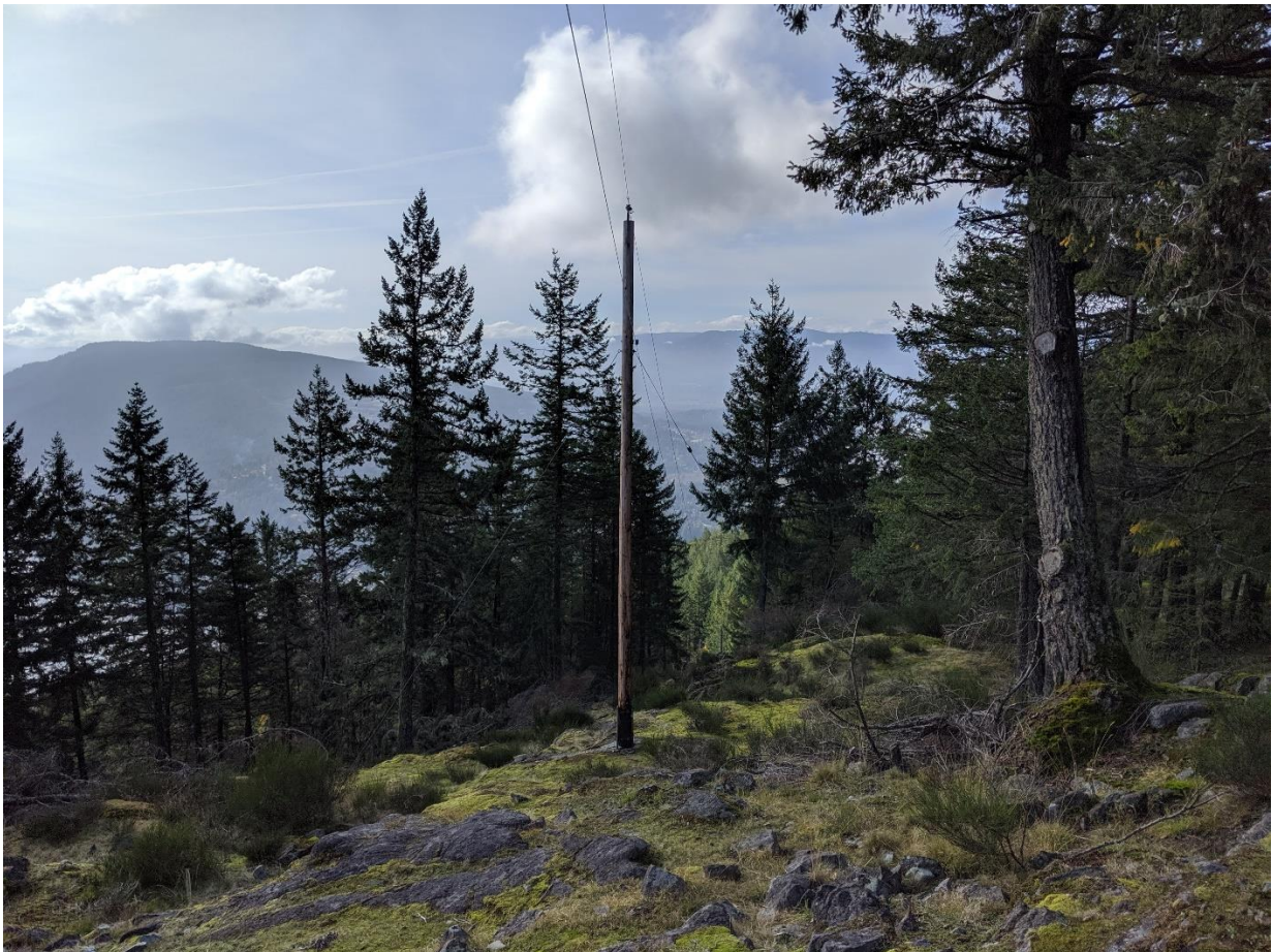
Photo 16: Power lines adjacent to forests are sources of ignition if trees or branches fall onto the lines.
