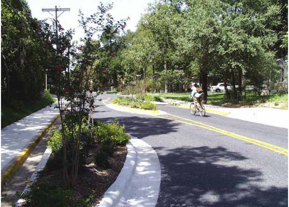
Chicanes calm traffic by narrowing vehicular lane widths and altering the street geometry
