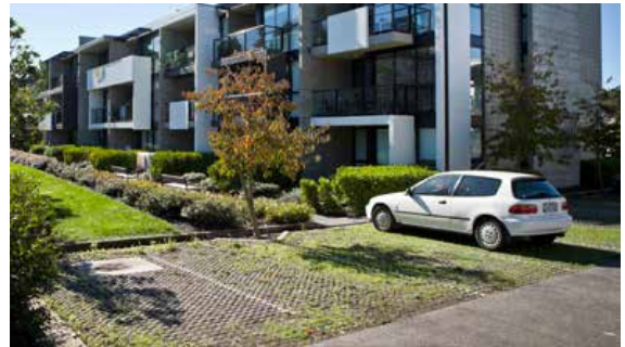
Permeable paving in a surface parking lot
