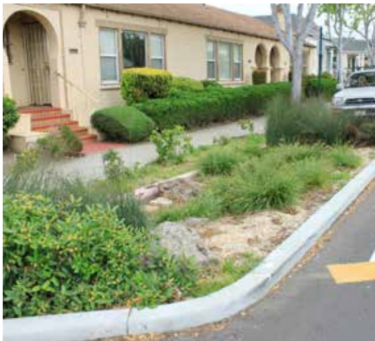
Stormwater swale interspersed with on-street parkingW
