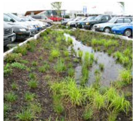
An on-site raingarden receiving parking lot run-off
