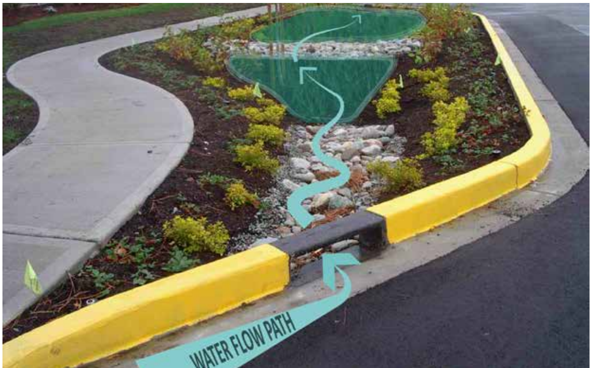
Stormwater flow path into on-street raingarden
