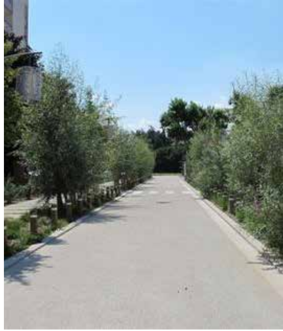
Shared space street with multi-functional landscaping
