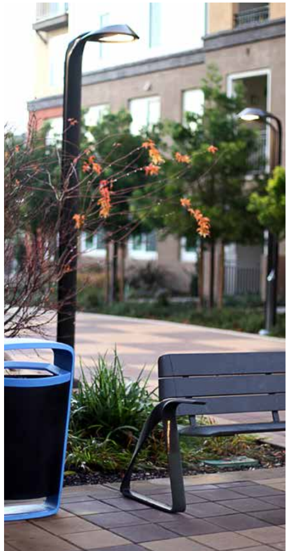
High quality streetscape with underground utilities and dark sky lighting
