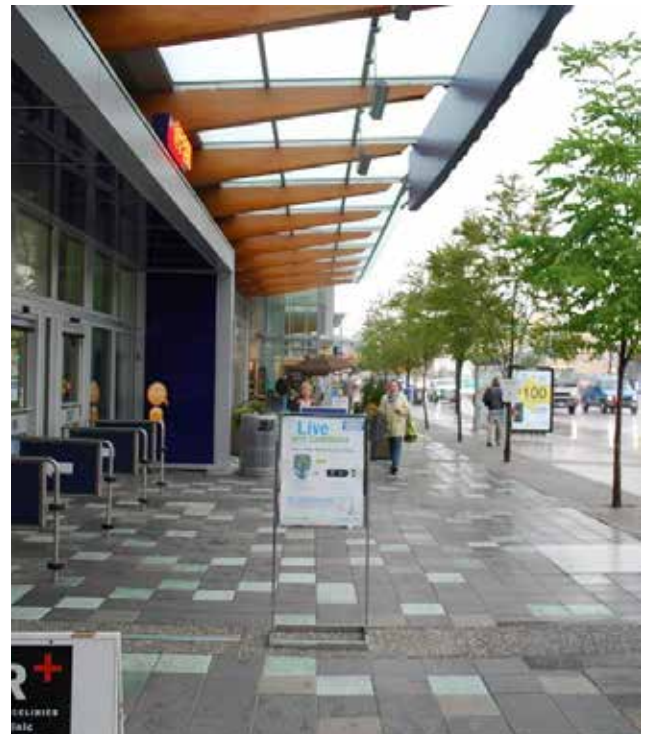
Building overhang providing weather protection
