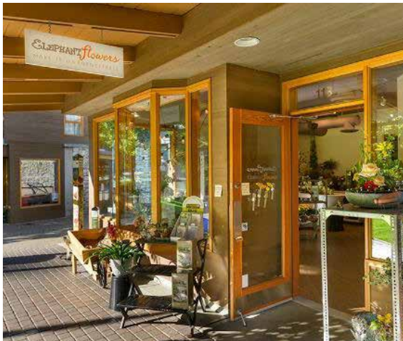
High quality build materials and architecture
