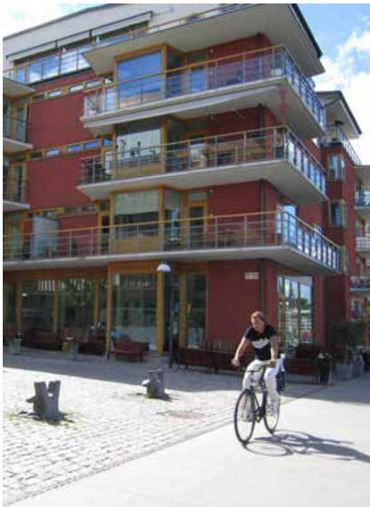
Residential balconies on upper storey units
