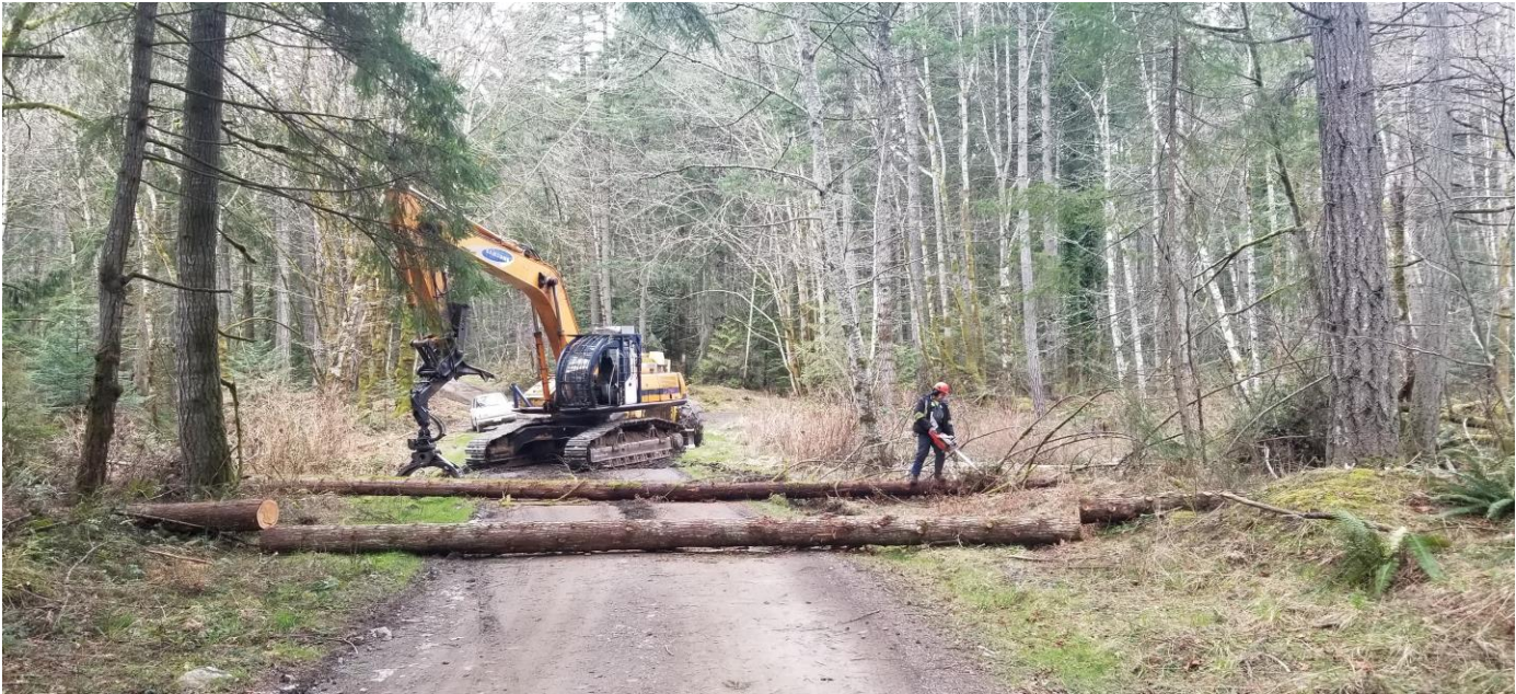
Mount Richards roadside salvage harvesting, removing blowdown and tree hazards from the roadsides.
