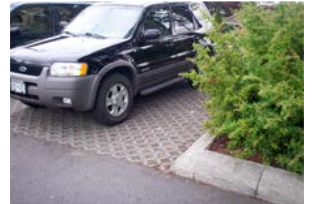
Example of permeous paving to reduce stormwater runoff
