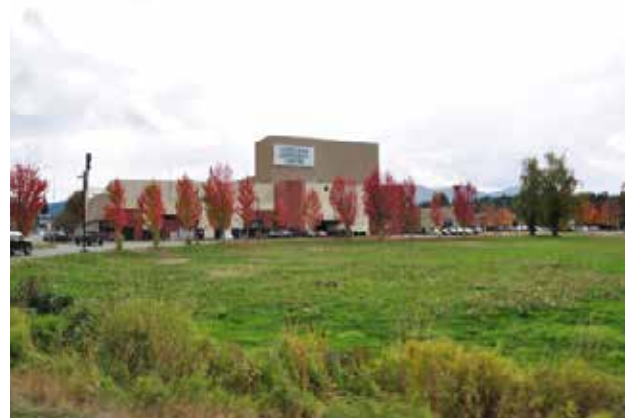
Figure 3.10: Cowichan Community Centre.
