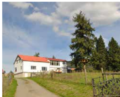
Figure 3.18: Existing rural residence.
