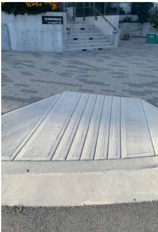
Figure 4.8: Curb Cut with tactile pavers for visually impaired.
